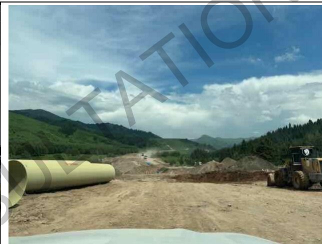
Photo 39: Ski resort access road and penstock for Jyrgalang HPP construction
