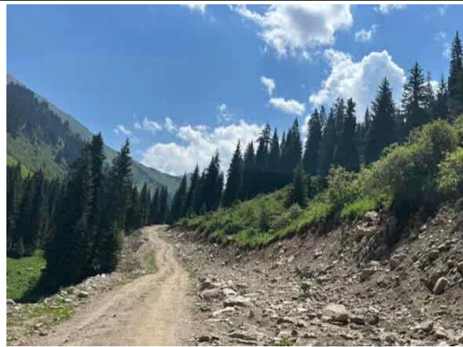
Photo 8: Road to intake, improved by project and with penstock on right hand side
