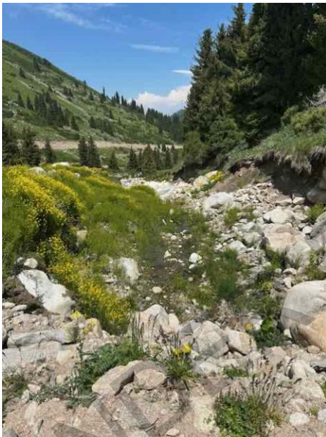
Photo 10: Former diversion channel
