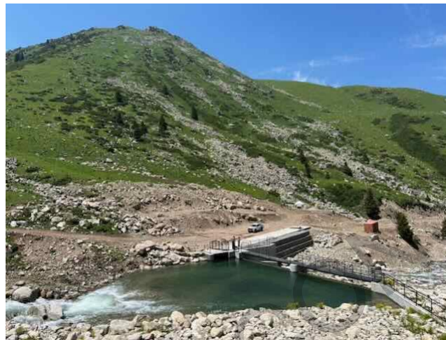
Photo 2: Boz-Uchuk HPP headworks area
