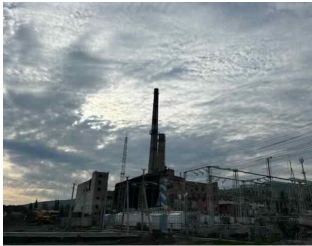
Photo 43: Defunct coal power and heating plant in Karakol
