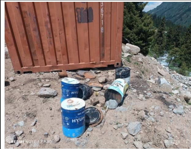
Photo 7: Water quality risks from materials not yet cleaned up at intake
