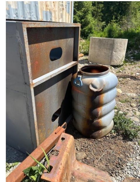
Photo 12: Construction materials to be cleaned up at powerhouse
