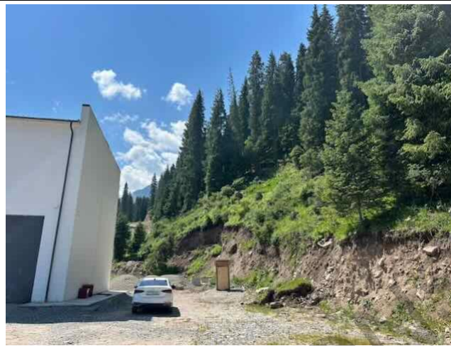
Photo 14: Area to the right of powerhouse with latrine, retaining wall to be built
