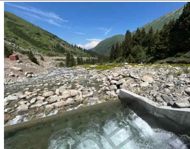
Photo 4: View downstream from spillway
