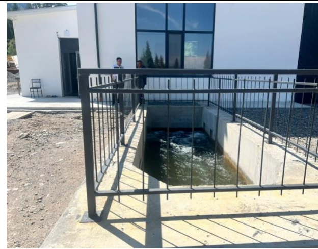
Photo 25: Tailrace channel from powerhouse
